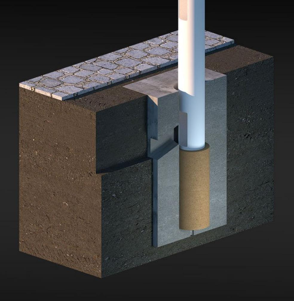
Thicken in fine sand. This will secure the Main Post in final position.
